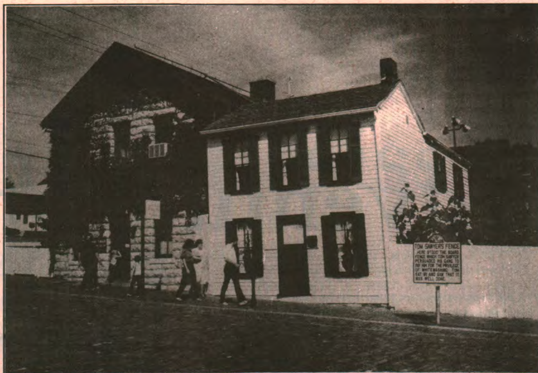
The small clapboard house on Hill Street was built in 1844 and is currently undergoing renovation.
